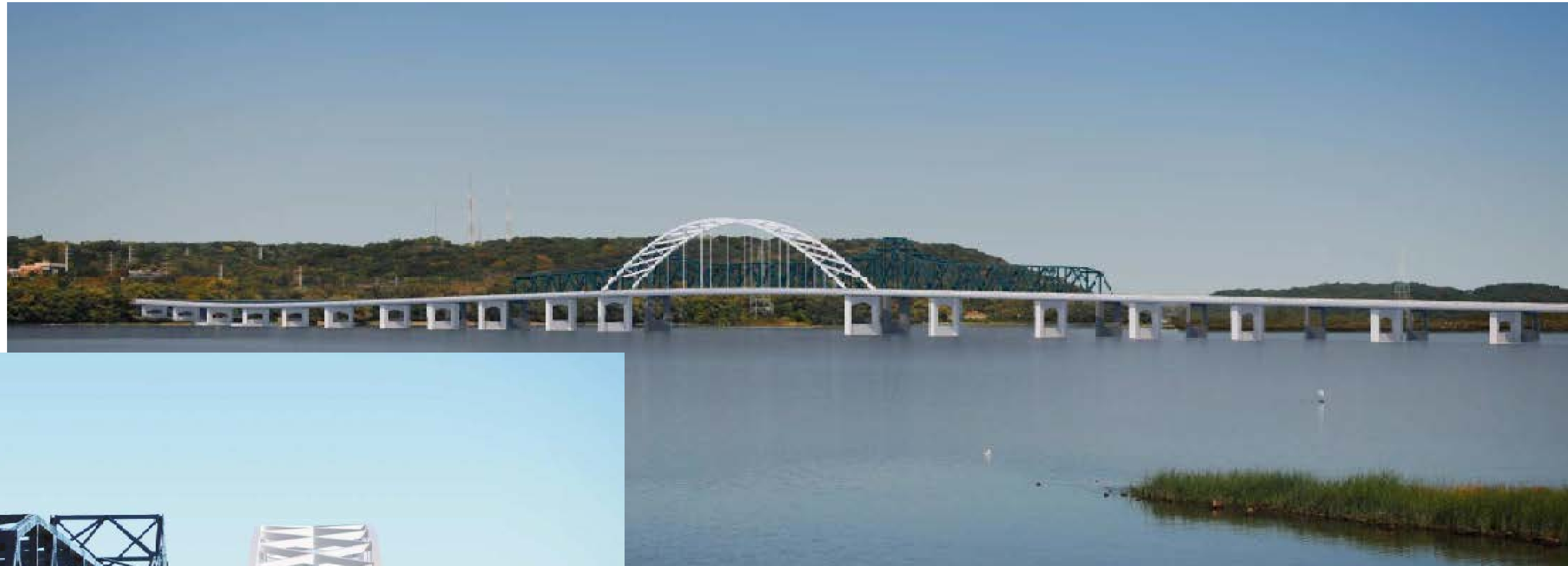
Southern View of Proposed Bridge Looking North
